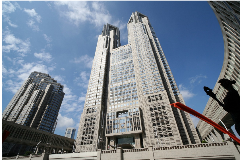
Figure 5: Twelve QuakeSaver sensors are installed in the Tokio Metropolitan Government Building by RISE partners at National Research Institute for Earth Science and Disaster Resilience (NIED).
